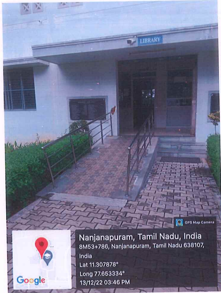
Ramps & Rails Located at Library Entrance
