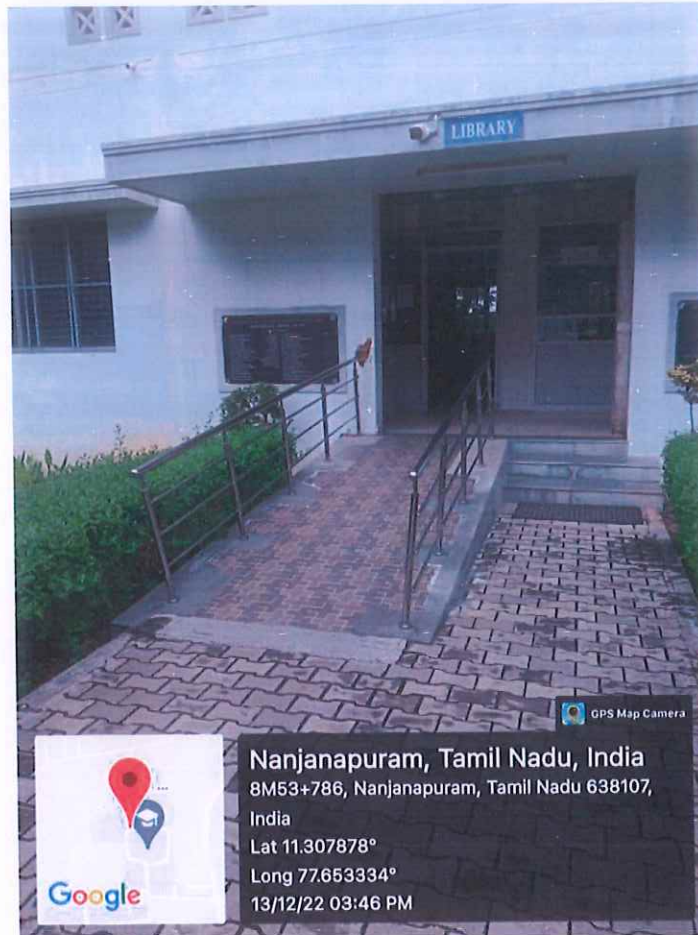
Ramps & Rails Located at Library Entrance
